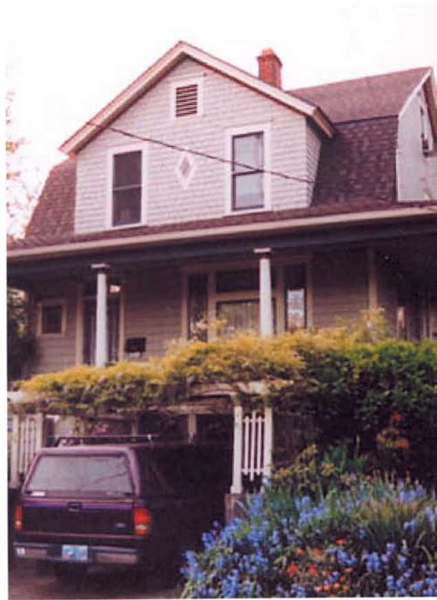
A charming wrap-around porch was uncovered during the remodel of Freitag's 1909 Dutch Colonial
